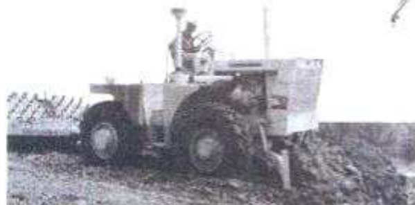
Spreading Fill, Pulling Compaction Rollers
