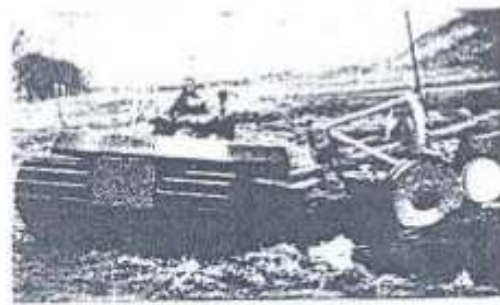
Ploughing 2ft. drainage channels.
